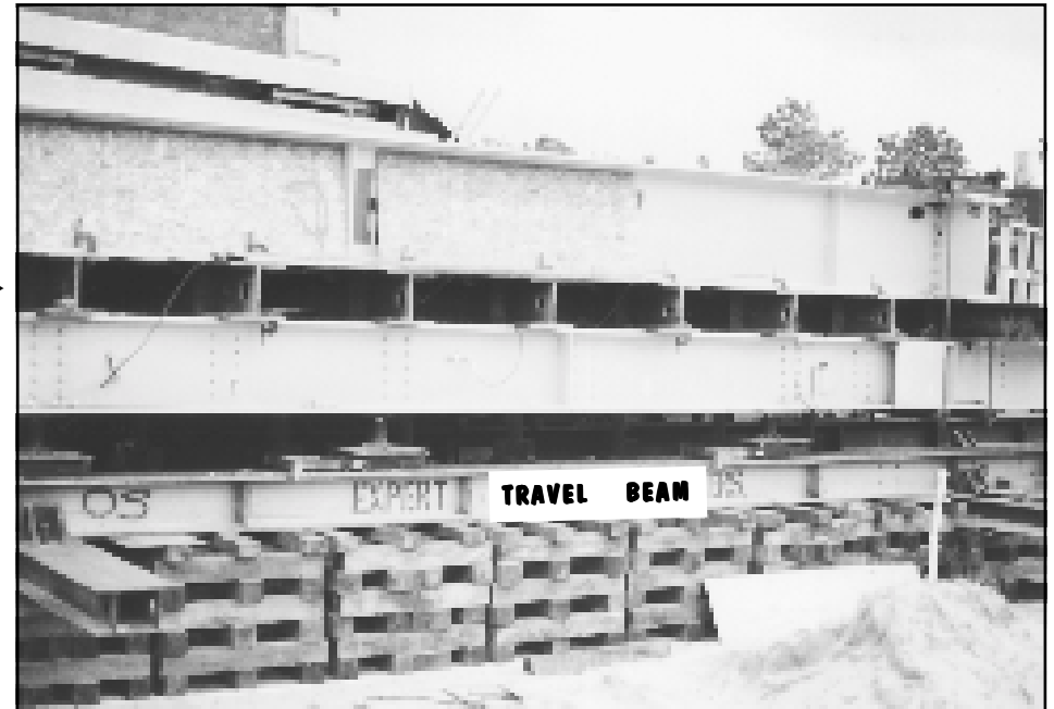
▶ Figure 23. Side view of unit (Note concrete under cribbing).
