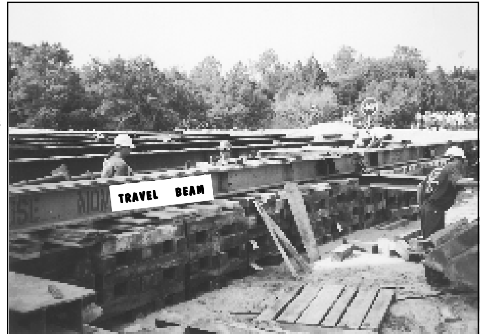
▶ Figure 19. Getting travel beams ready for final push.
