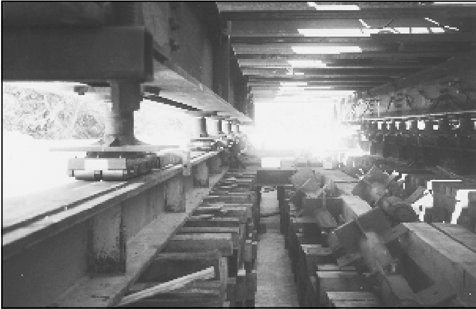
▲ Figure 25. Lifting red cylinders prepared for roller/travel beam jack removal.
