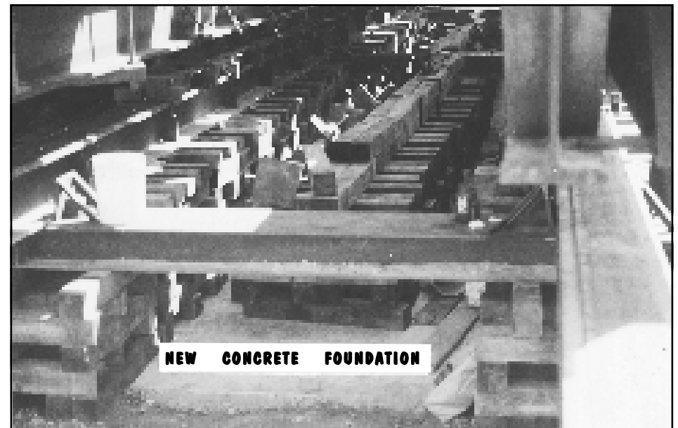
▶ Figure 21. Underneath view showing cribbing on new concrete foundation.
