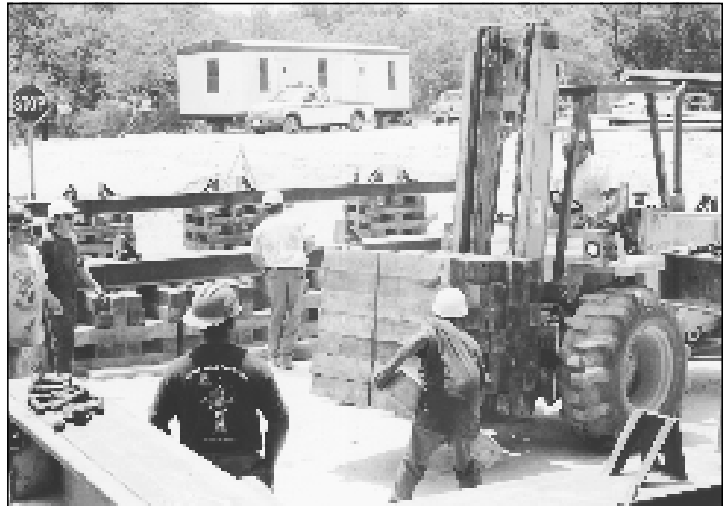
Figure 18. Forklift with pile of cribbing for placement of final travel beams.
