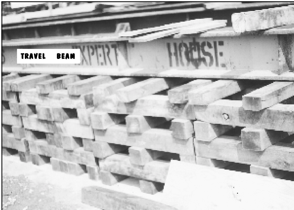
▼ Figure 20. Cribbing over concrete foundation (Note travel beam).
