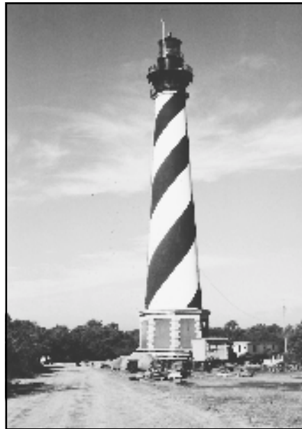
▲ Figure 27. Lighthouse in final location for lowering onto concrete foundation.
