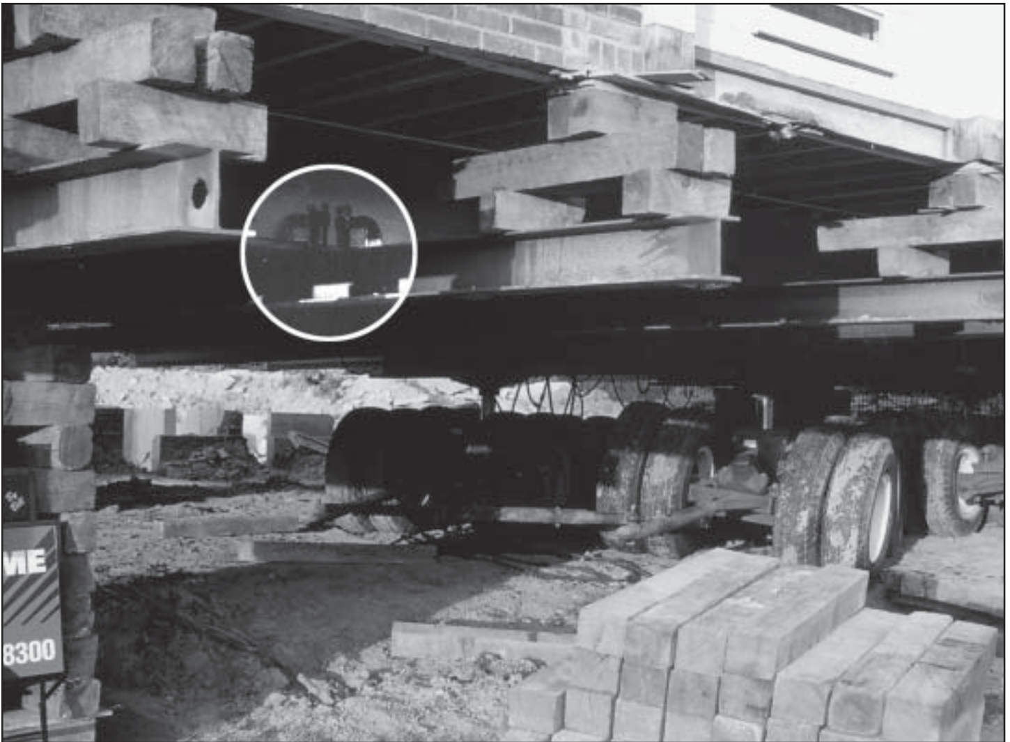
C-clamps were used to hold cross loaders to the main beams.
