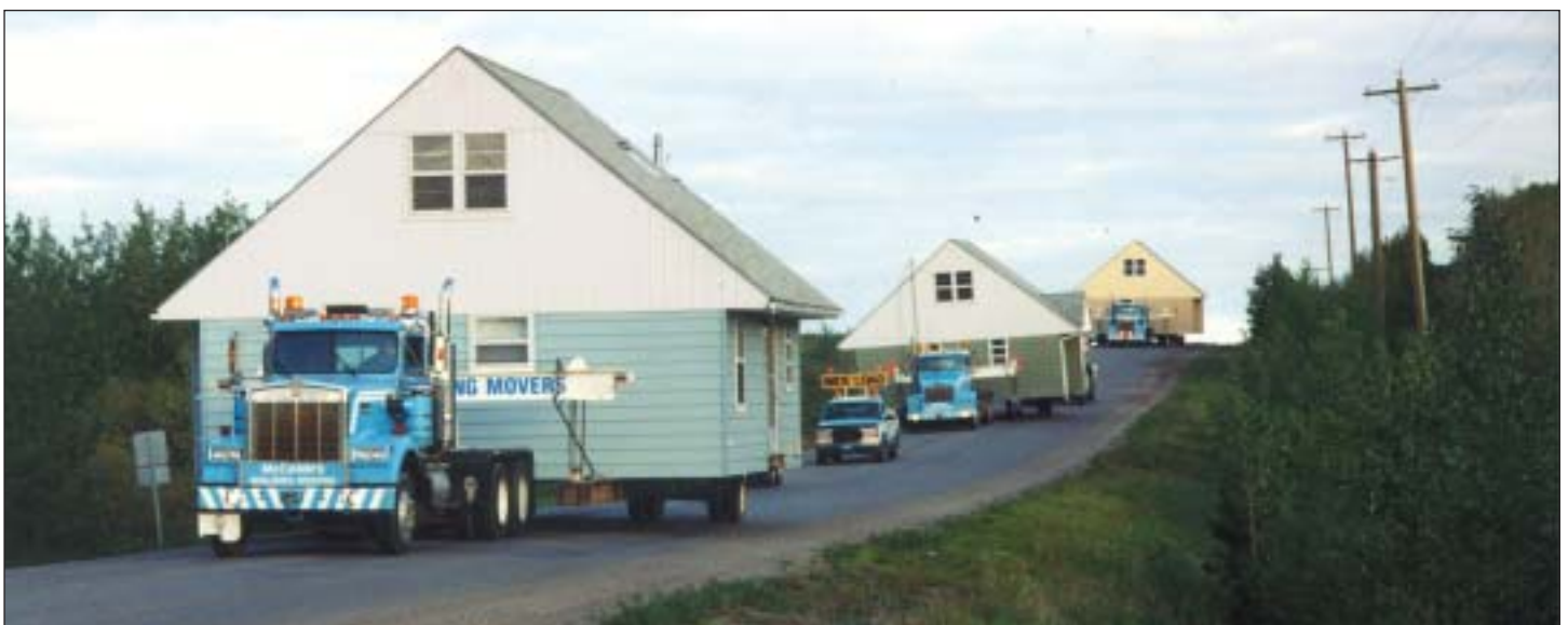
Three of twelve army barracks in Calgary being moved to the Sik Sika Indian Reservation. The buildings were stored on blocks through the winter and placed on basements the following spring.
