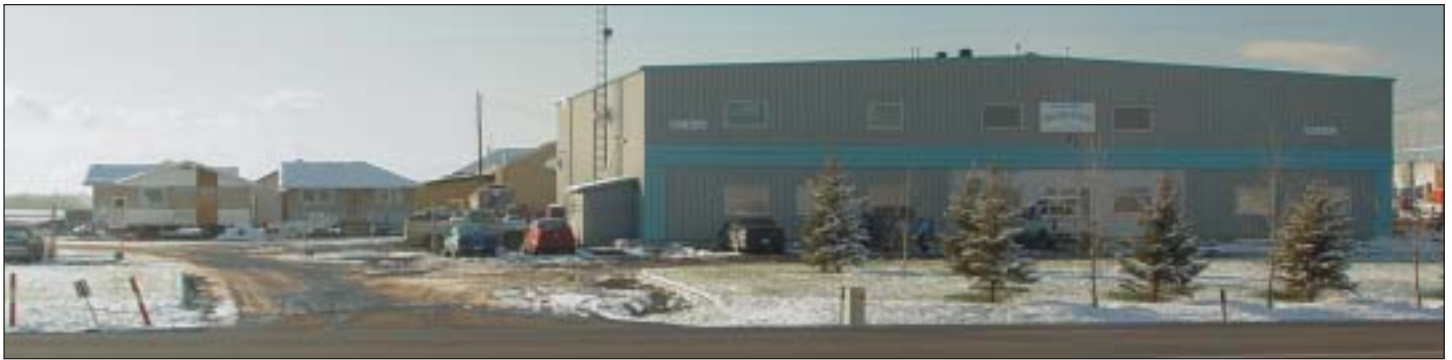
The company's current headquarters in Calgary.
