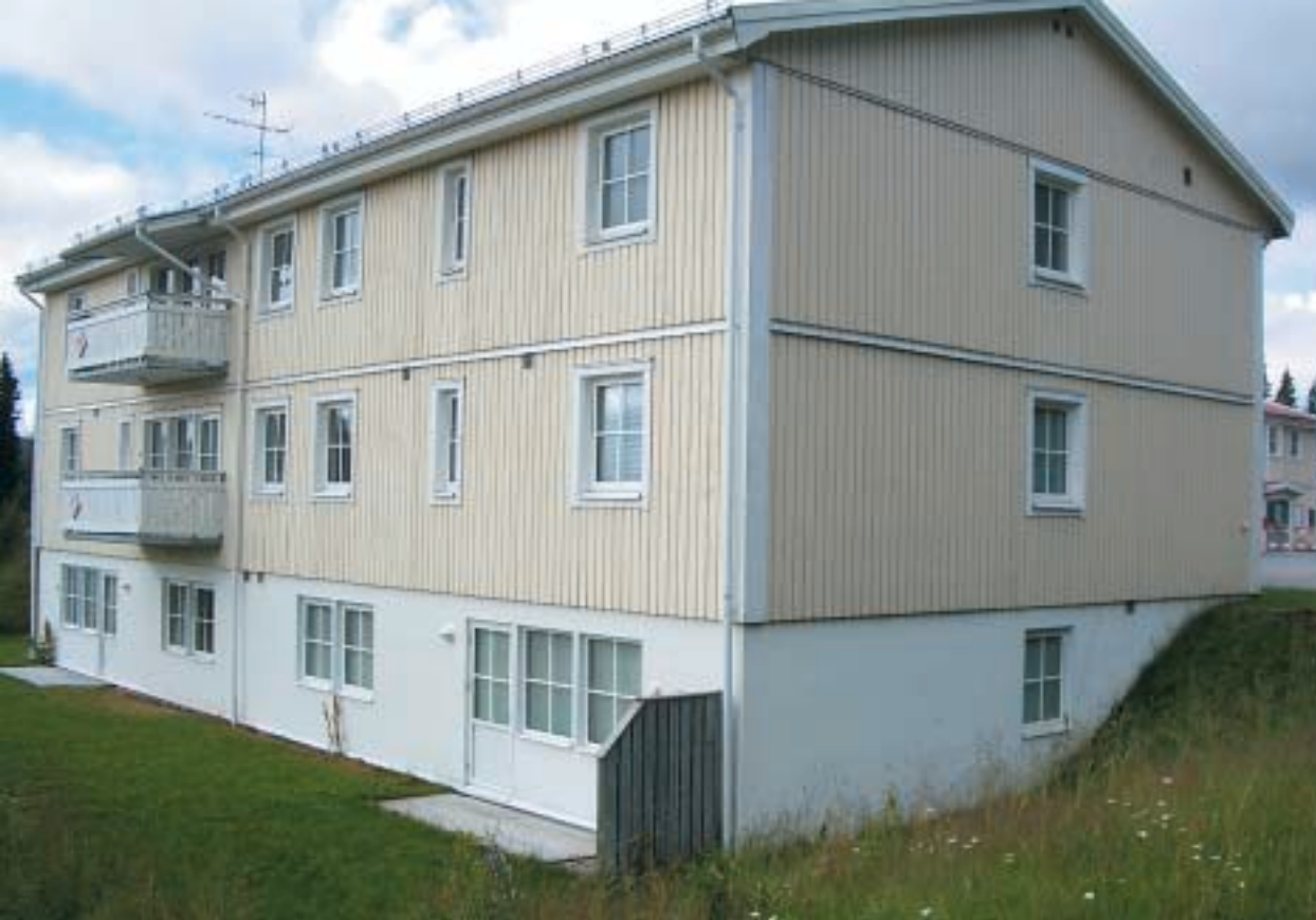
The building before the work started.
