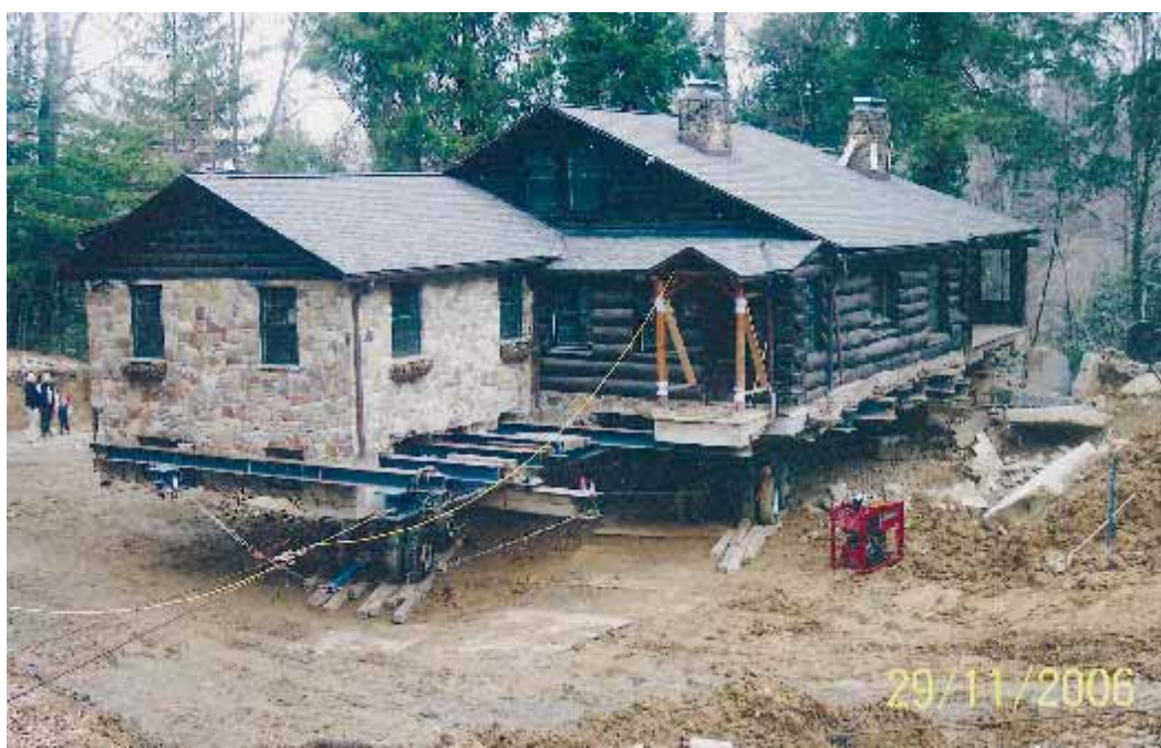
This Stafford Log Cabin in Gates Mills, OH was 80-feet x 40-feet with stone walls and was moved on the same site in 2006. Rain and muddy conditions made the move almost impossible. The owner eventually was required to excavate one-foot of soil at the new location and add one-foot of limestone fill. The structure was moved due to severe erosion.
