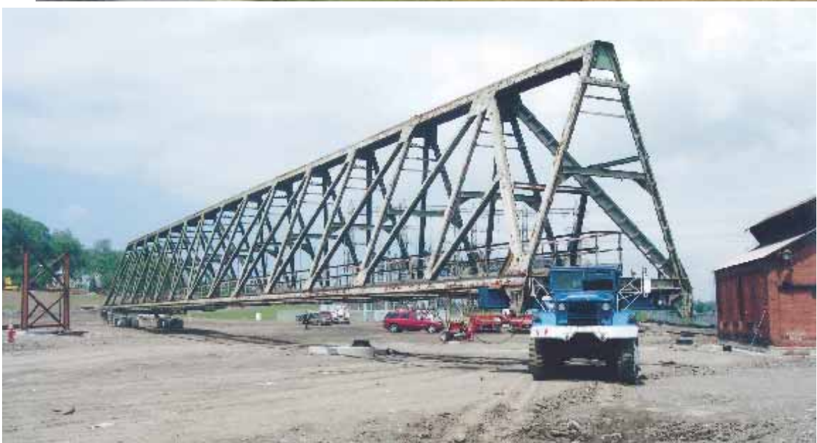
A 500-ton brick and stone train station with a concrete floor in LaFayette, Indiana was moved five blocks to a new site in 1994.
