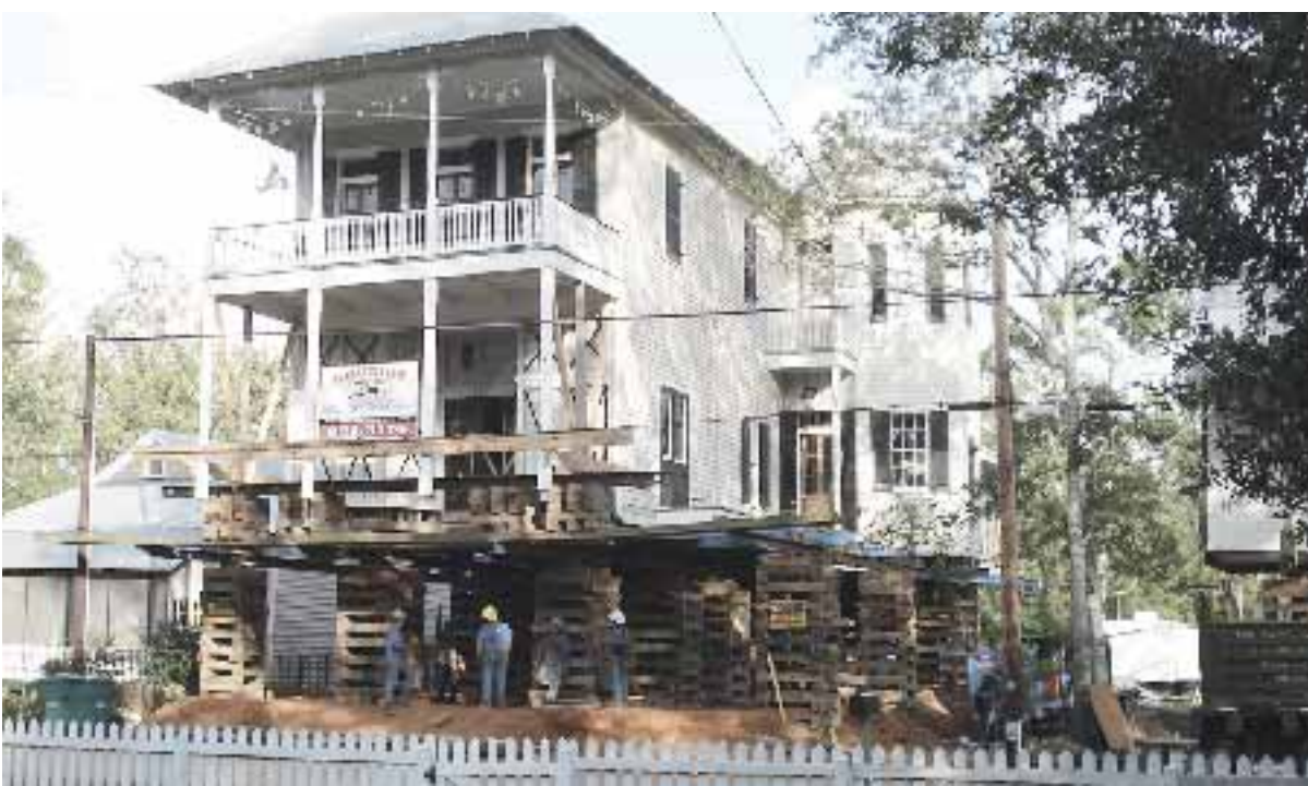
Roubion Construction contracted with IASM member DeVillier House Movers and Leveling to elevate both structures.
