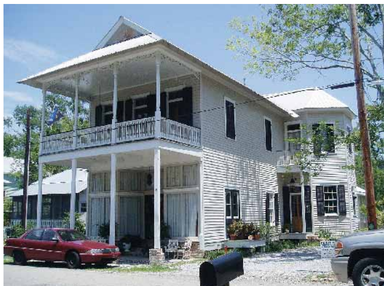
The main residence before elevation began.
