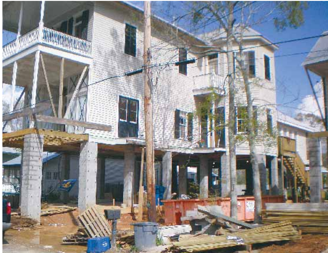
Frontal view of the main residence after installation of piers.
