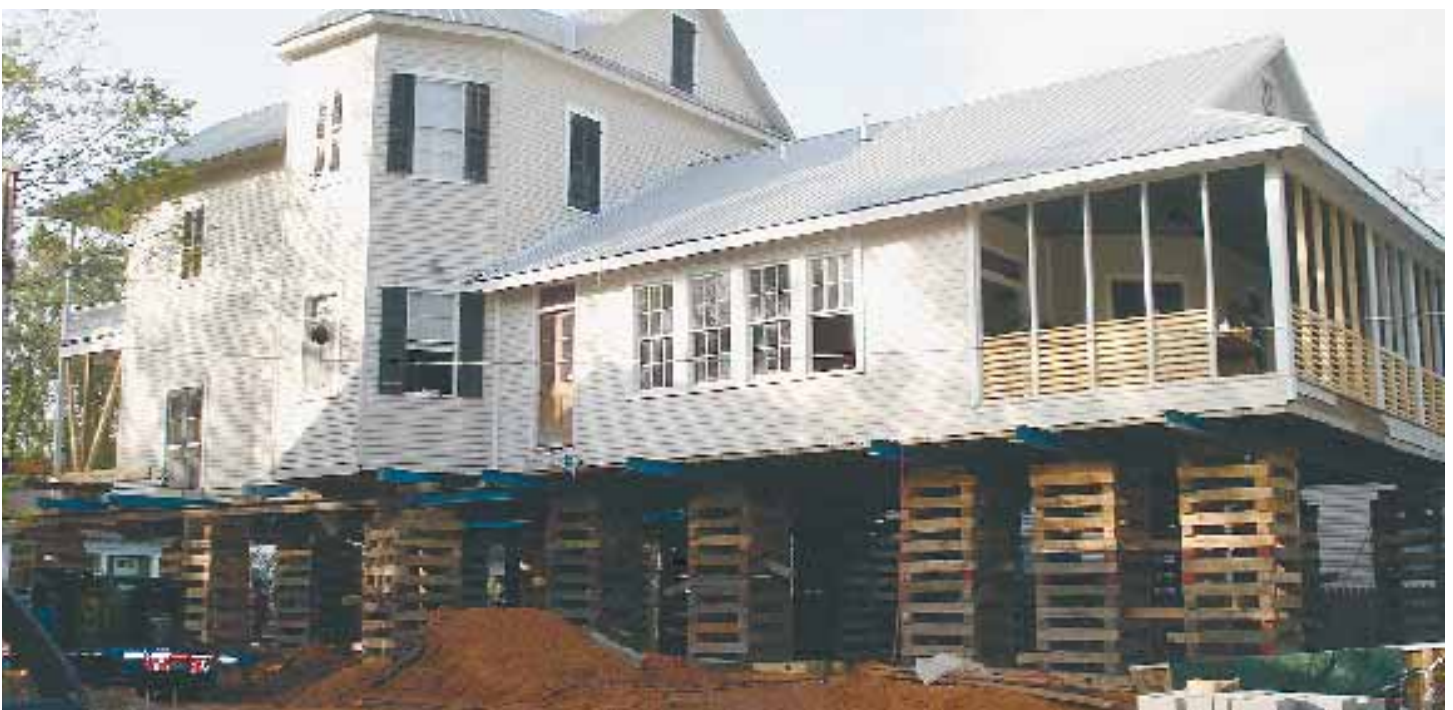
(Below) Cribbing for the second lift.
