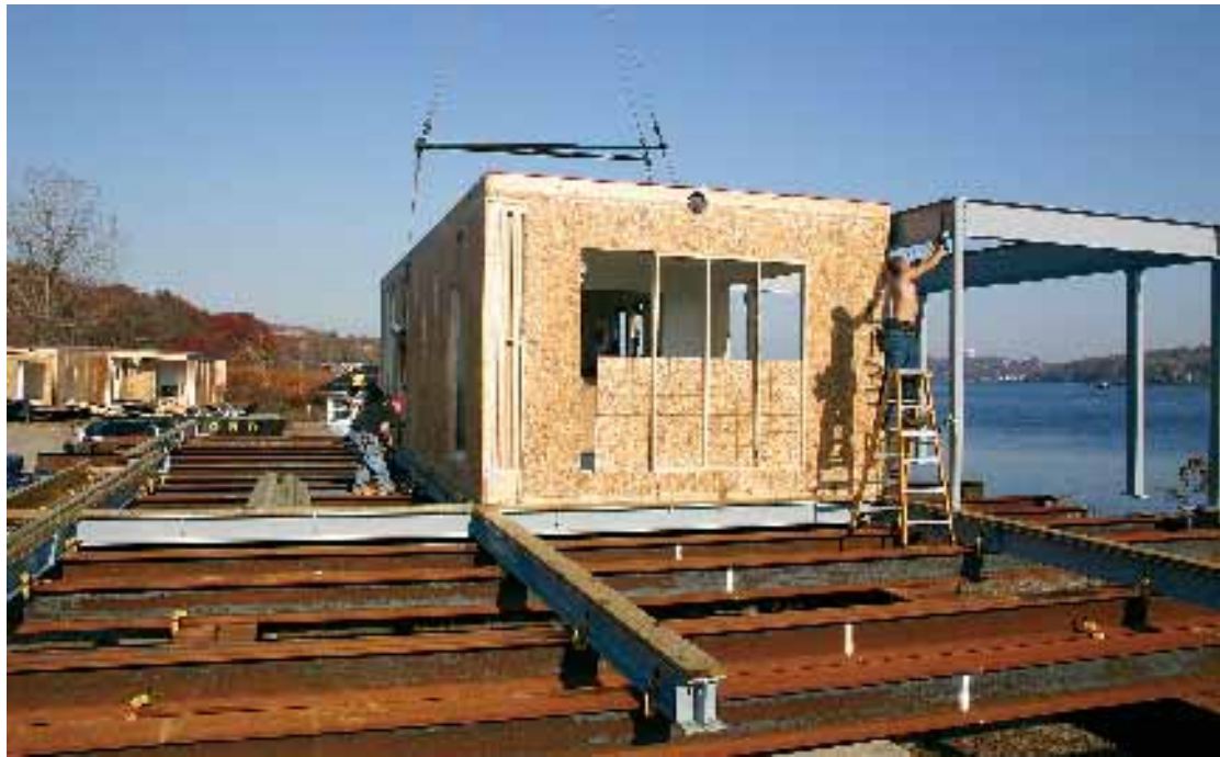
The custom house was constructed to a finished level on steel at a temporary jobsite in New London, CT
