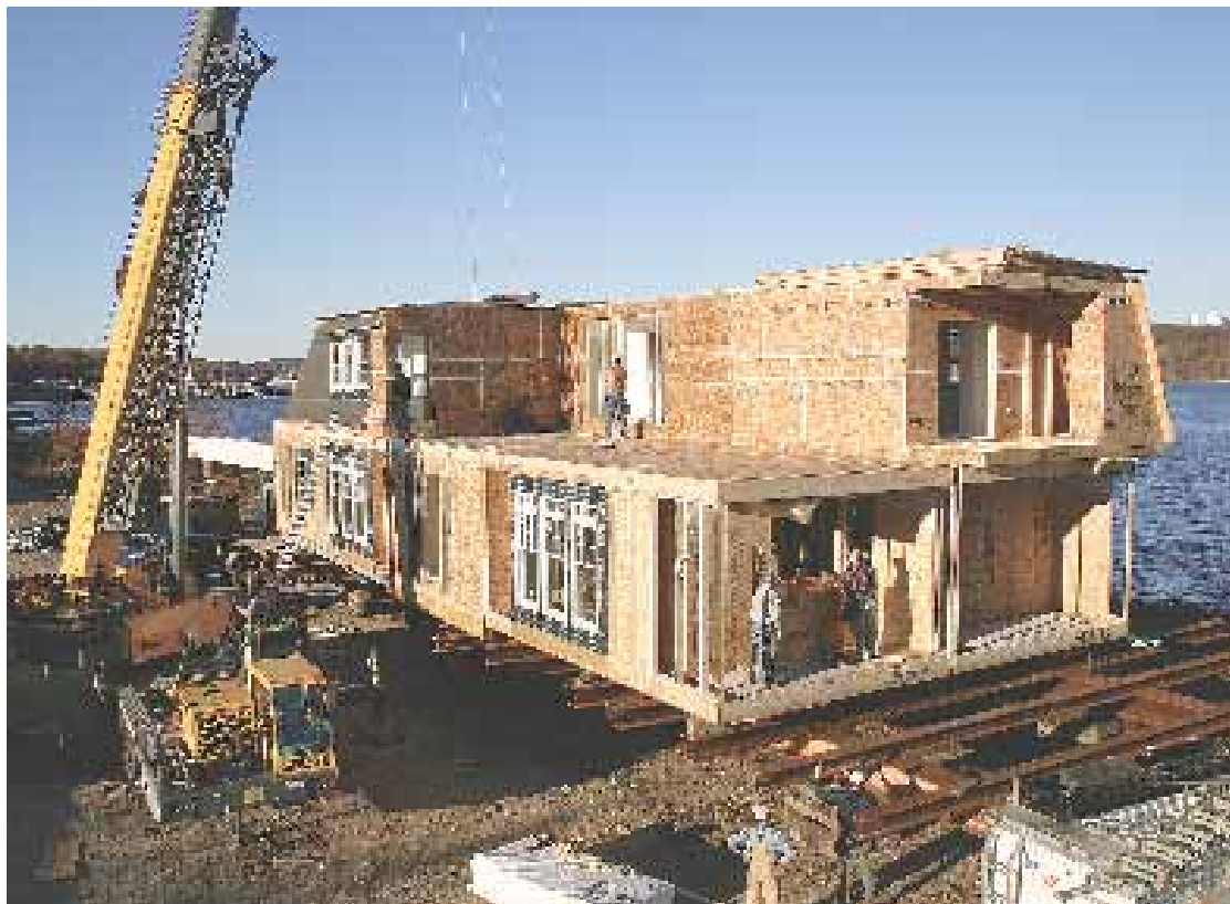
The custom house was constructed to a finished level on steel at a temporary jobsite in New London, CT
