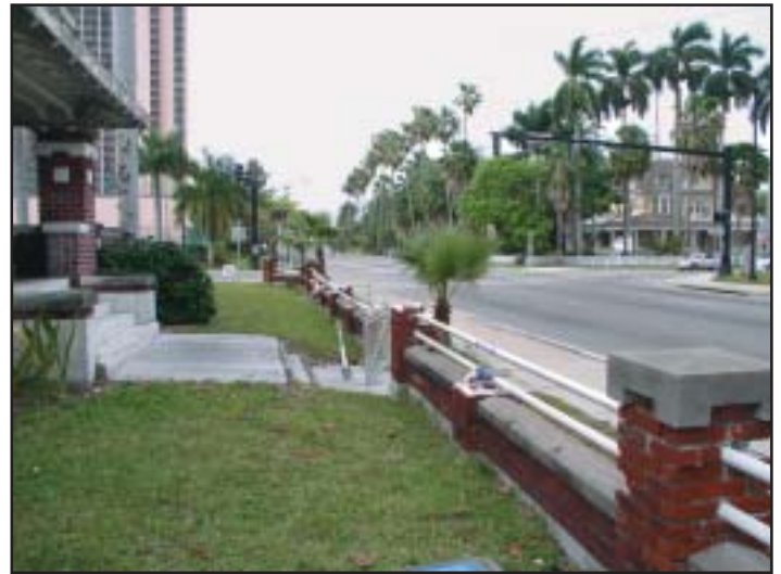
Even though much clearing was required before the structure could be moved, the trip was a short one—just across the street.
