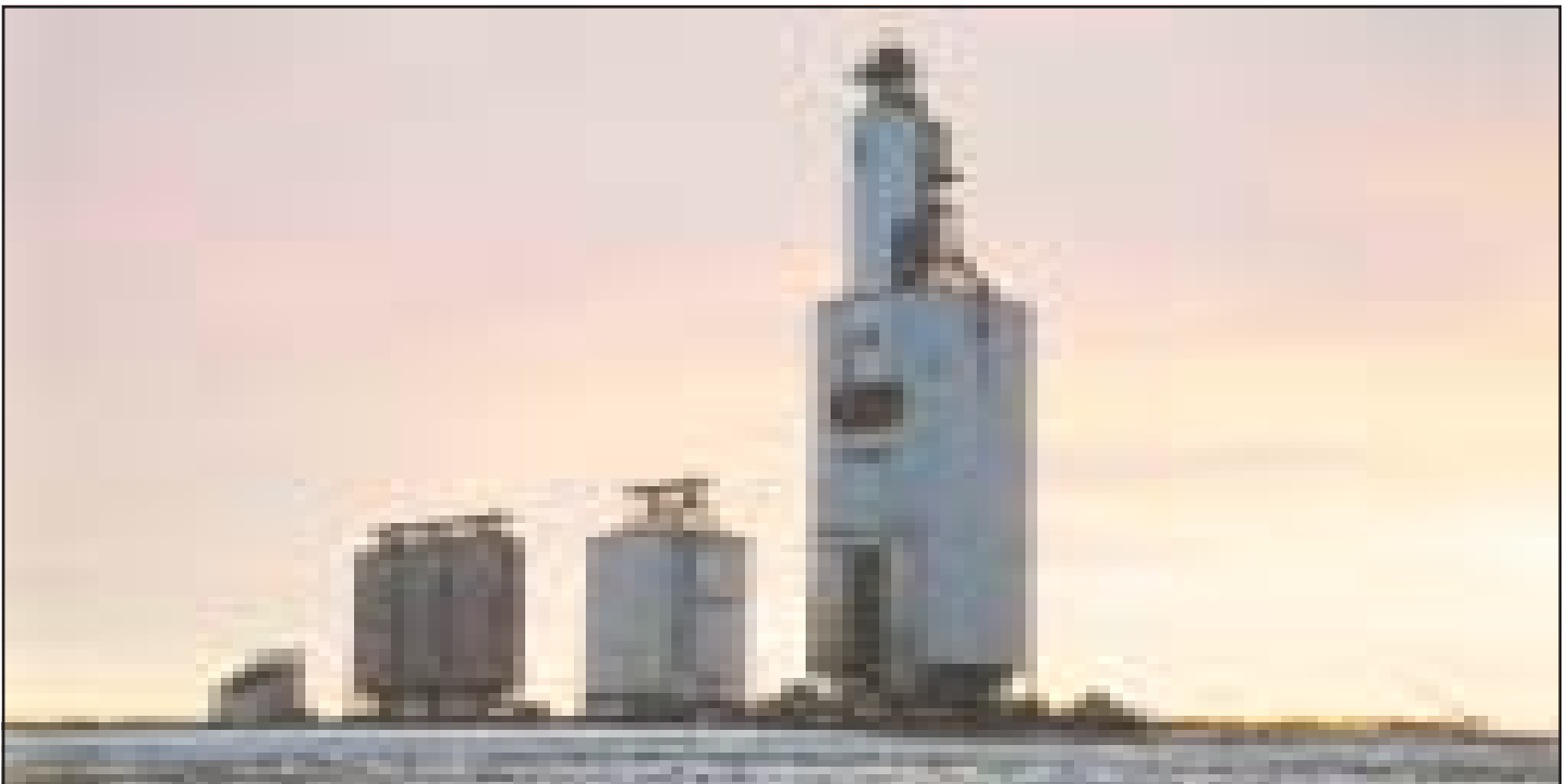
Four structures were transported at the same time in order to reduce the cost of elevating utility wires.
