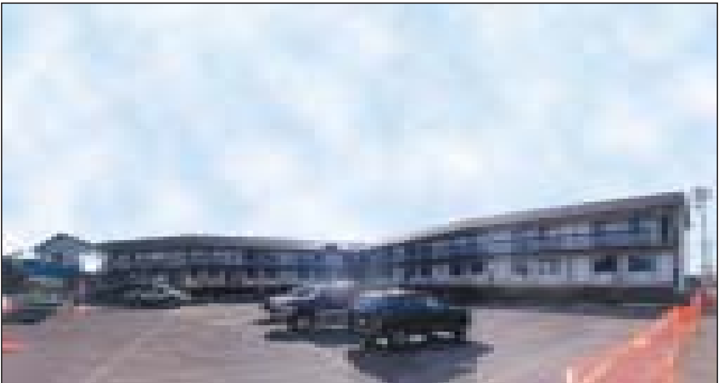
The 42 units motel that weighed 500 plus tons was raised three feet and one inch in one lift.
