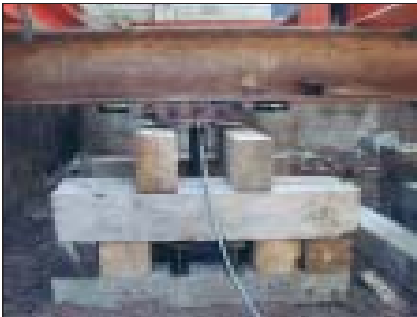
This innovative moving technique used pressurized rollers.
