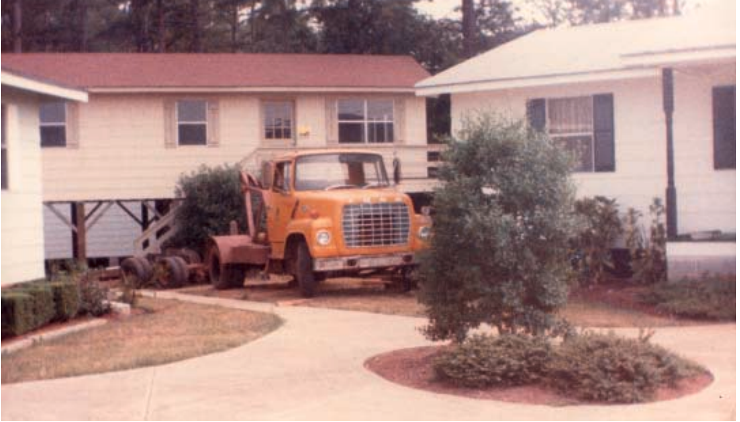
The first job performed by Coburn in the early 1980's was moving nine structures for Jim Walter Homes.
