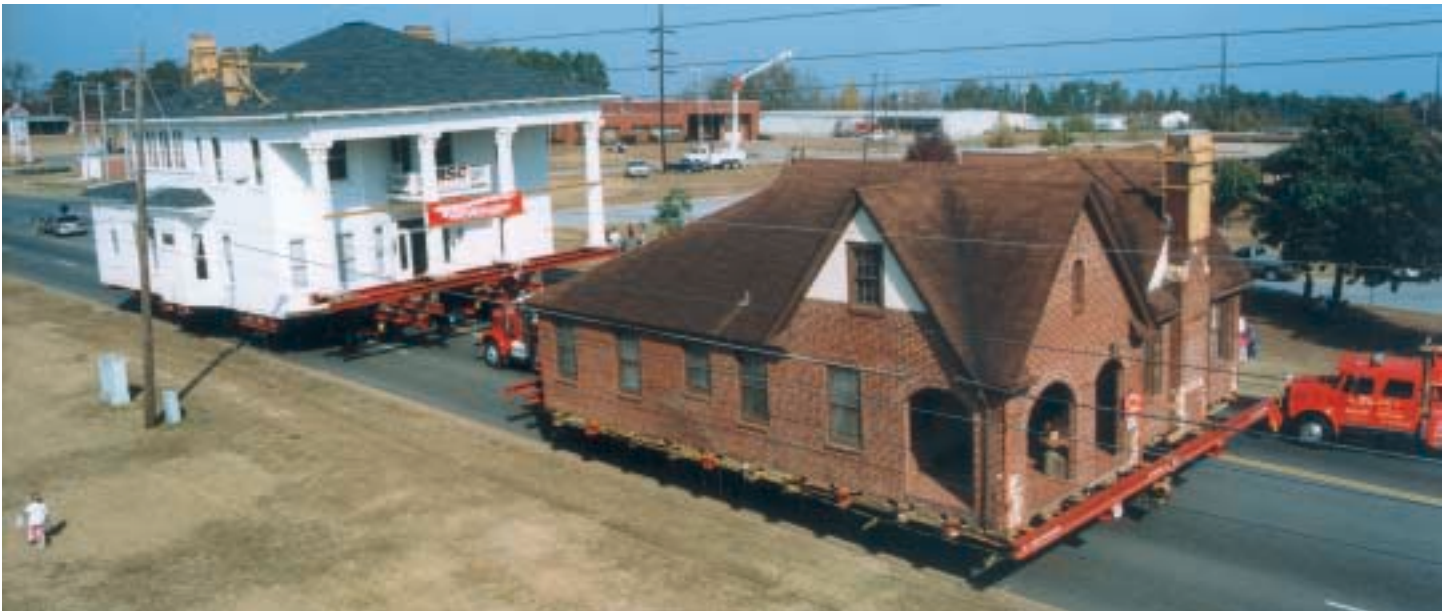
Two structures being moved simultaneously in Opelika, AL in 2001
