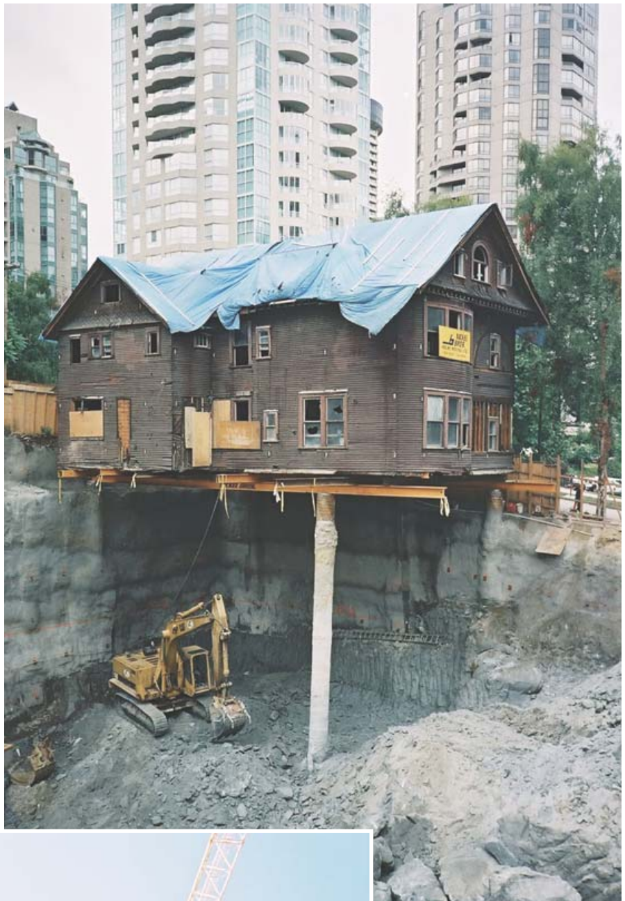
Building is in place on piers and caisson.
