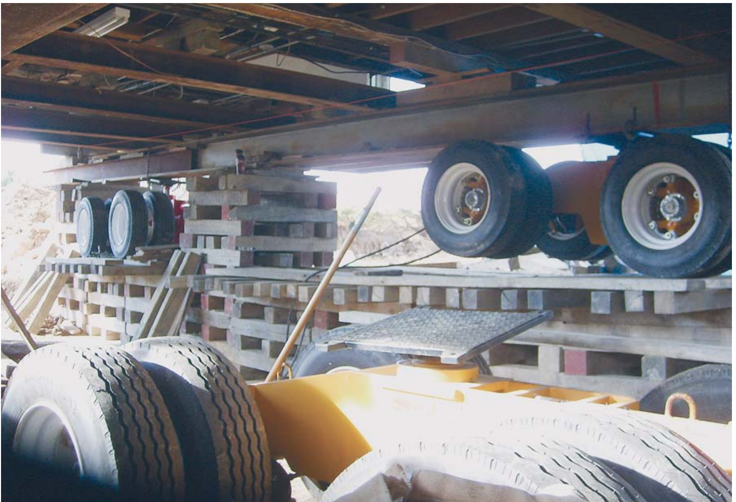
The day before the move, The Parish House was secured on four hydraulic dollies.
