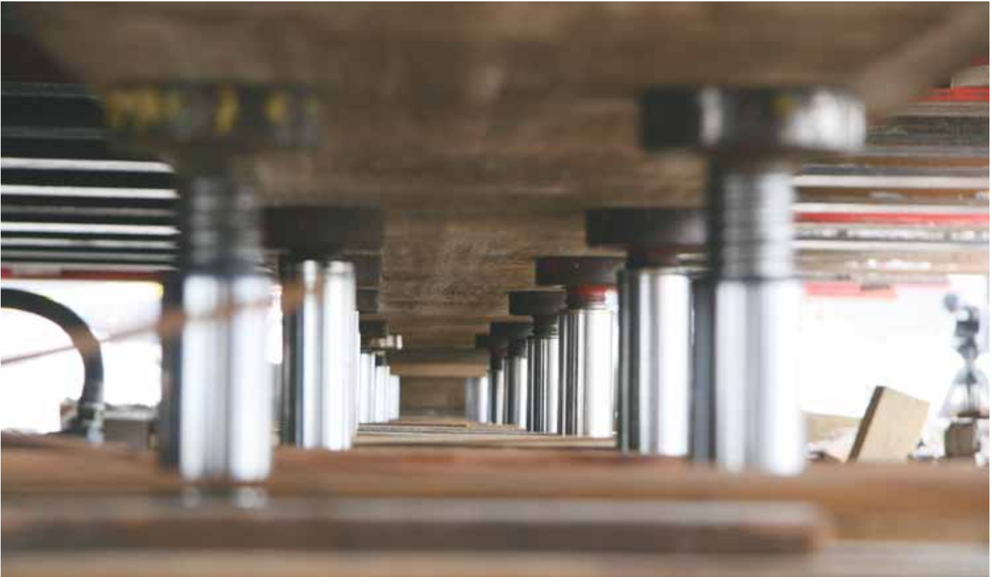
The structure was elevated 32 inches using a 24-jack unified jacking machine.
