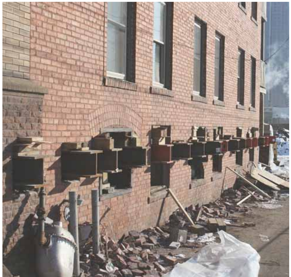
50-foot long cross beams were spaced at 42 inches.
