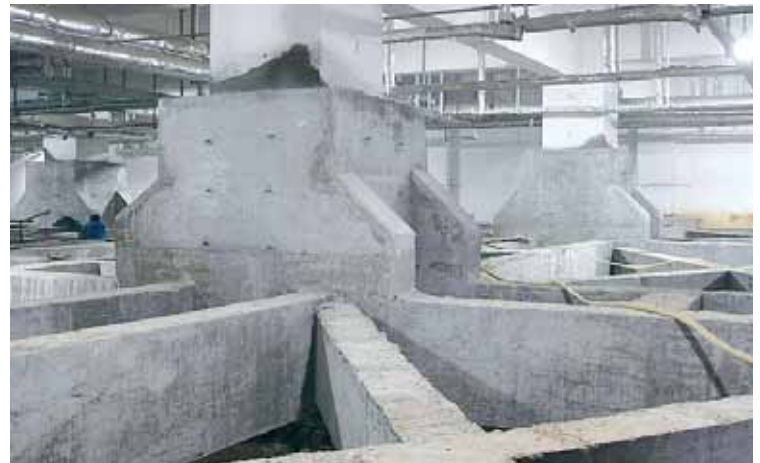
Lattice to strengthen between joints.
