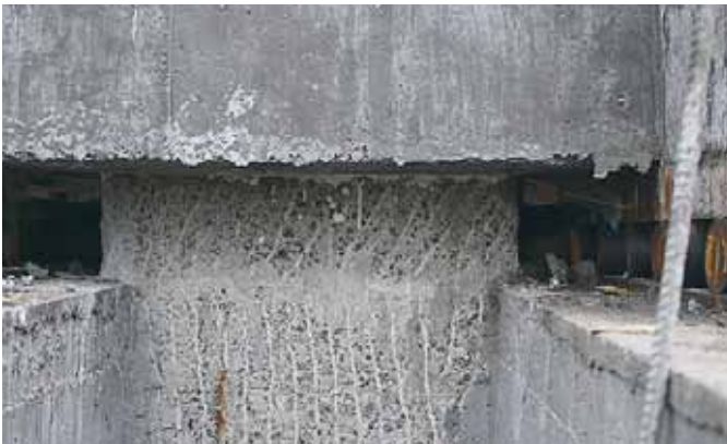
Column prior to cutting with rails cast each side.
