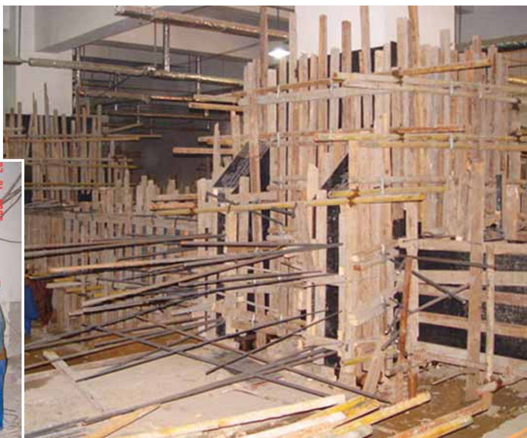
Formwork for columns.
