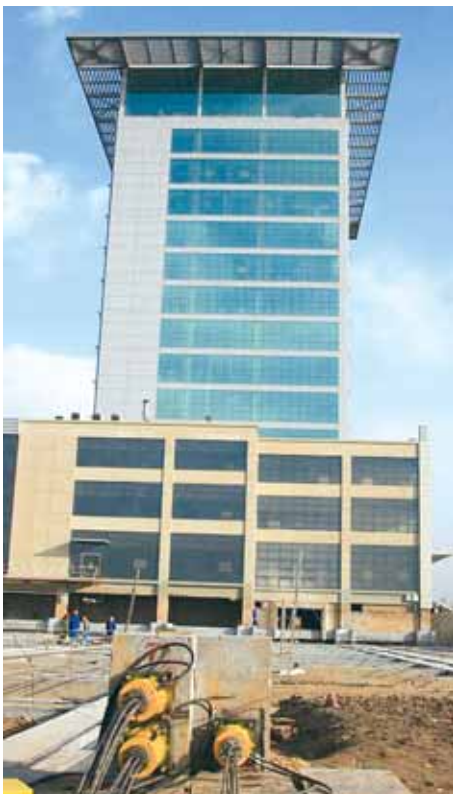
15-story building, Shandong Province
