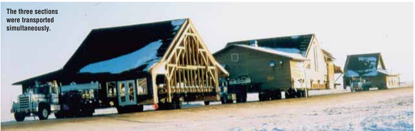
The loaded structure leaving the site by way of a cleared road across a field. This was necessary to preserve trees planted too close to allow the building sections to pass. A temporarily constructed wall is plainly in view.
