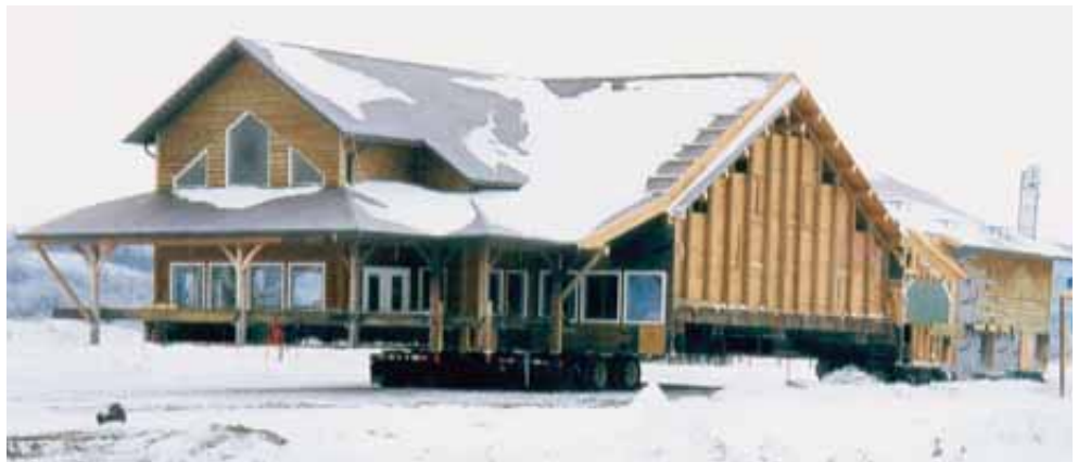
The loaded structure leaving the site by way of a cleared road across a field. This was necessary to preserve trees planted too close to allow the building sections to pass. A temporarily constructed wall is plainly in view.
