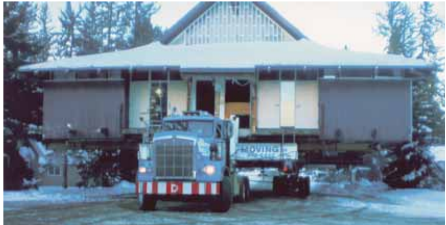
Major power lines and trees this corner to take four hours prior to parking for the night.
