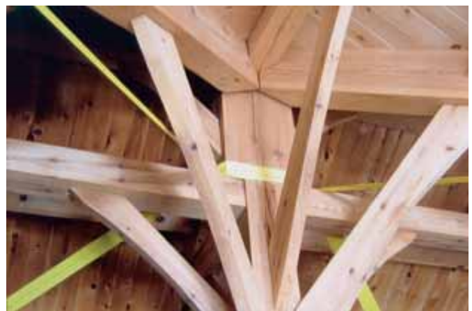
Bracing straps to minimize joint separation and cosmetic damage to wooden beams.
