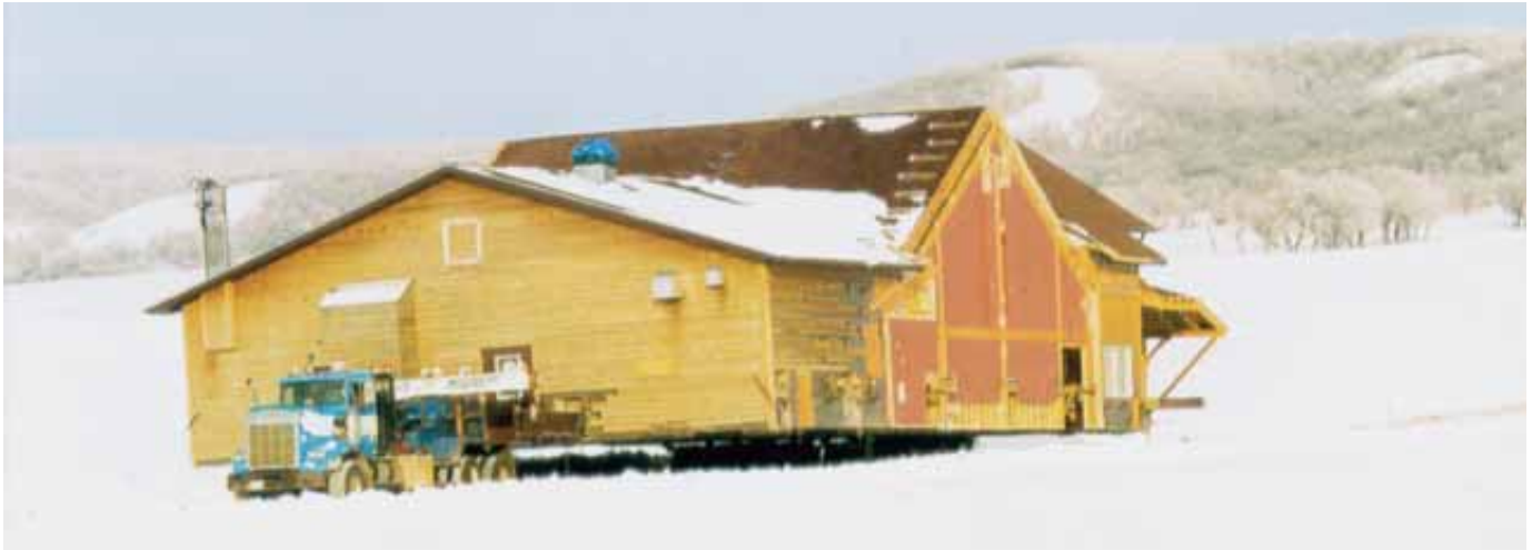
Even though the structure had been separated into three sections the loads were large as shown here, being pulled by a Kenworth.
