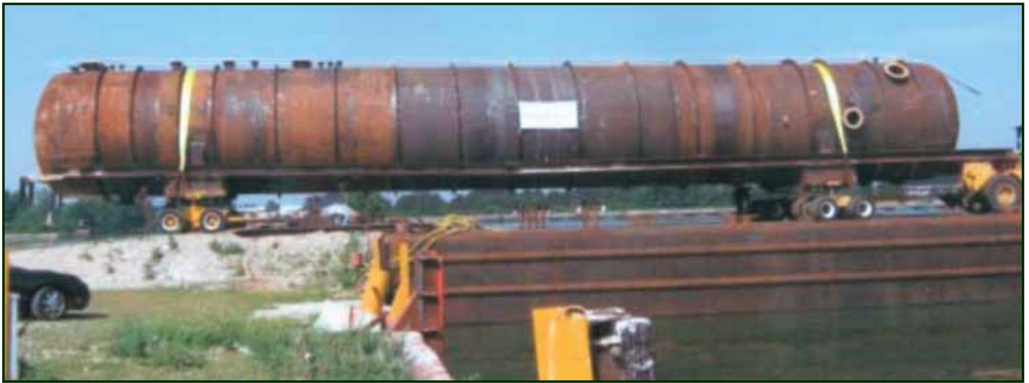
Loaded vessel up on dollies to achieve adequate ground clearance for loading onto the barge in Sandusky
