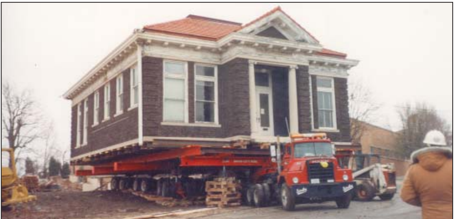
Moving a Carnegie Library in Mexico, MO in 1991.
