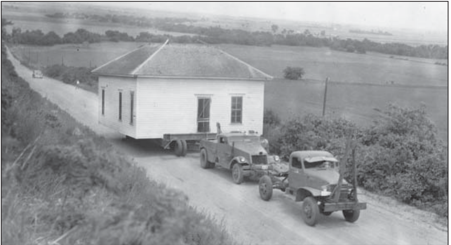
First house moved by the company in 1949 using two 1942 World War II Army trucks.
