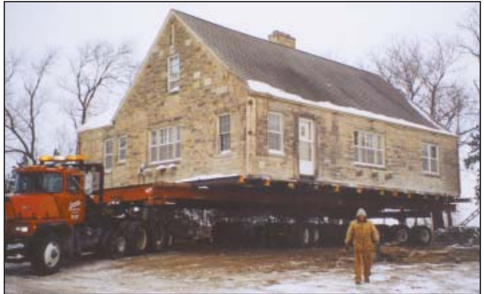
This stone house was moved in the Winter of 2004 in Lincoln, NE
