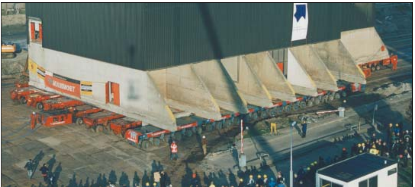
Once the building had reached the top of the 1% slope a short official starting ceremony was held witnessed by hundreds of guests and on-lookers.
