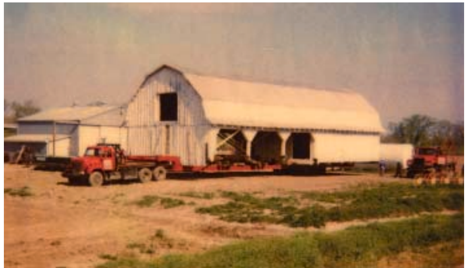
A 28' x 70' barn was moved on Leatherman Plantation in Tunica County, MS
