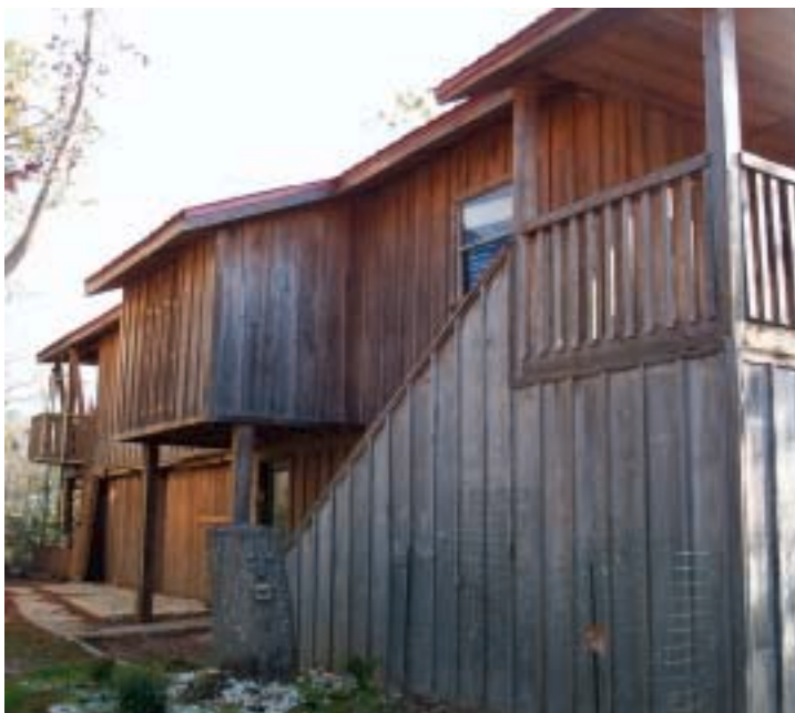
This 28' x 62' structure located near the Biloxi River was elevated from six to 11 feet. Before (left), After (right)
