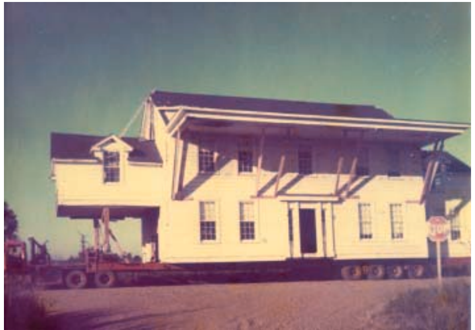
Moving a 32'x'90'two-story house in mid 1980's in Shelby, MS for Dr. Ming.
