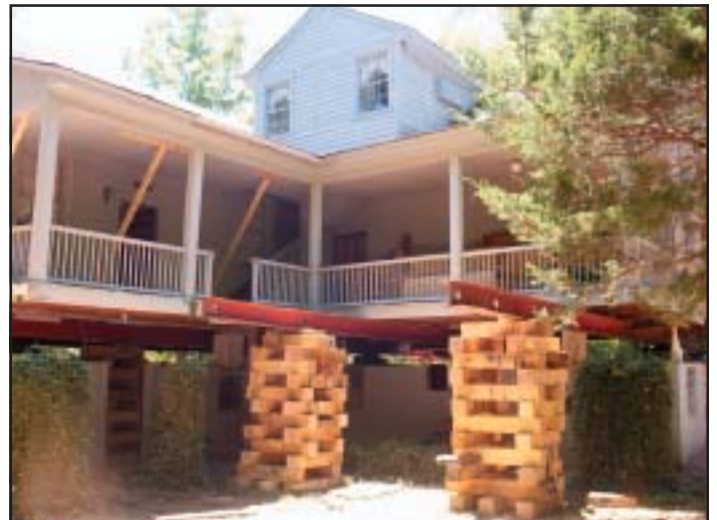
Moving a 32'x'90'two-story house in mid 1980's in Shelby, MS for Dr. Ming.
