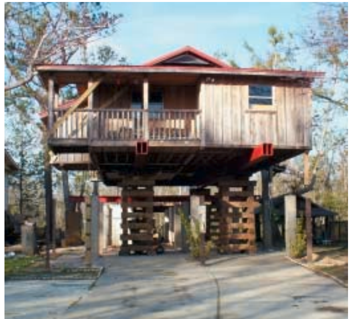
This 28' x 62' structure located near the Biloxi River was elevated from six to 11 feet. Before (left), After (right)
