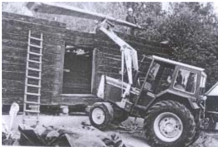
Tractor with loader used for dismantling
