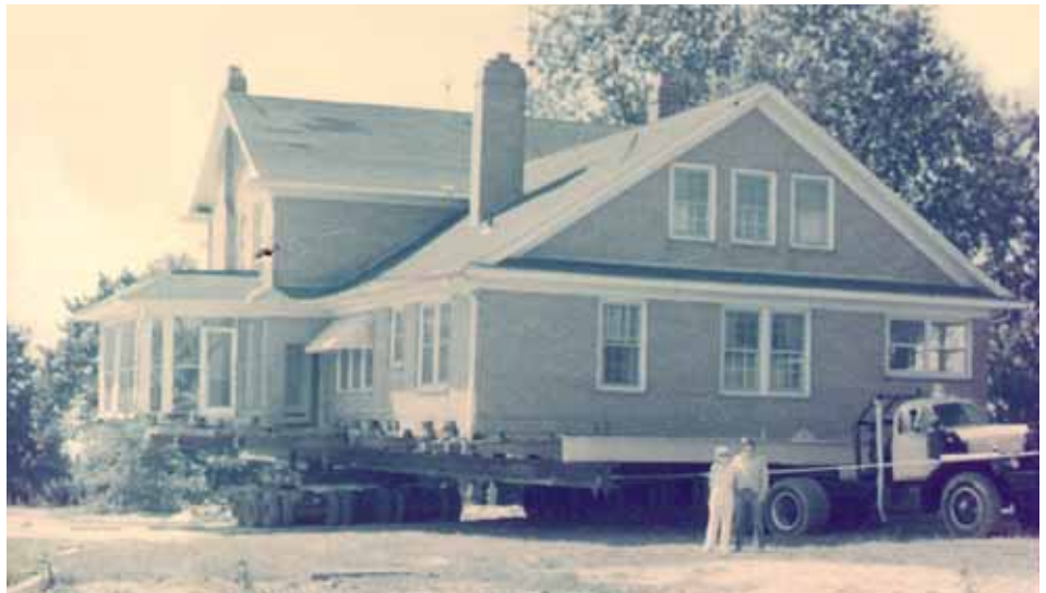
The 350-ton Blackwood House being relocated in Greensboro, NC in 1974.
