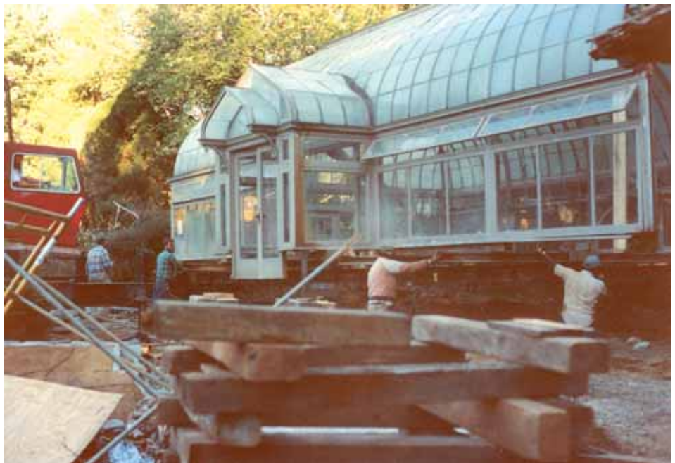
A glass and cast iron steel greenhouse on the Bowman Gray Estate was relocated in 1982.
