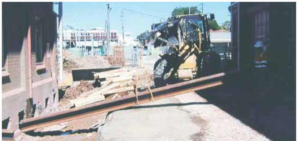
Installation of cross beams showing excavation limit due to underground cables.
