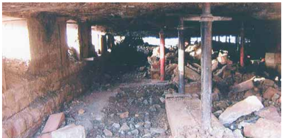
Partition wall footers and windows cut in perimeter wall.
