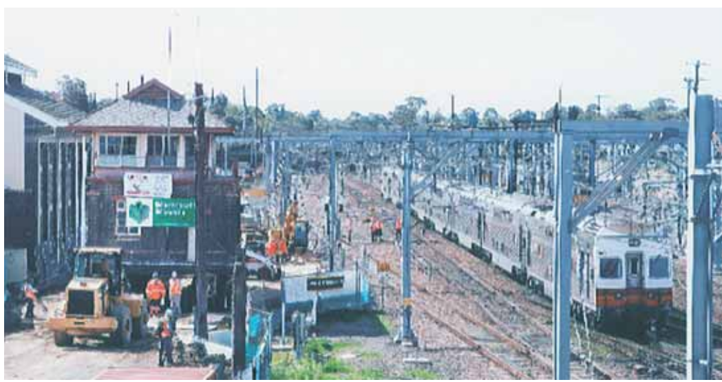
Halfway along its relocation path showing adjacent rail lines.
