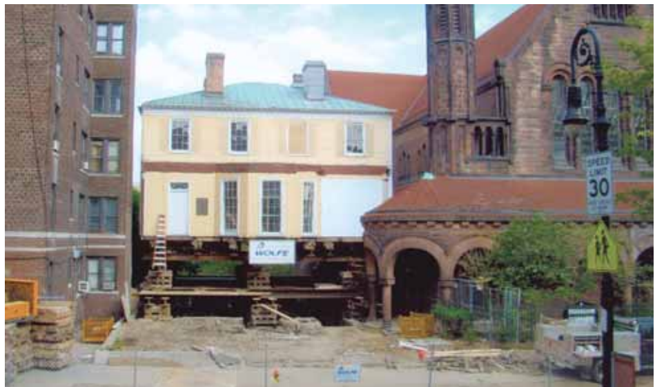
View from the street as the Grange is lifted. It needs to clear the rounded portico on the right
