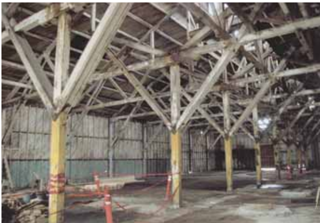
Interior view of the shed showing unique truss structure.
