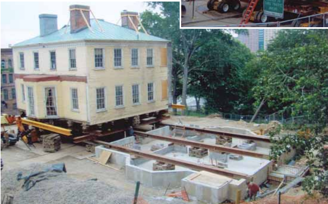
Preparing to skate the Grange overtop the new foundation.
