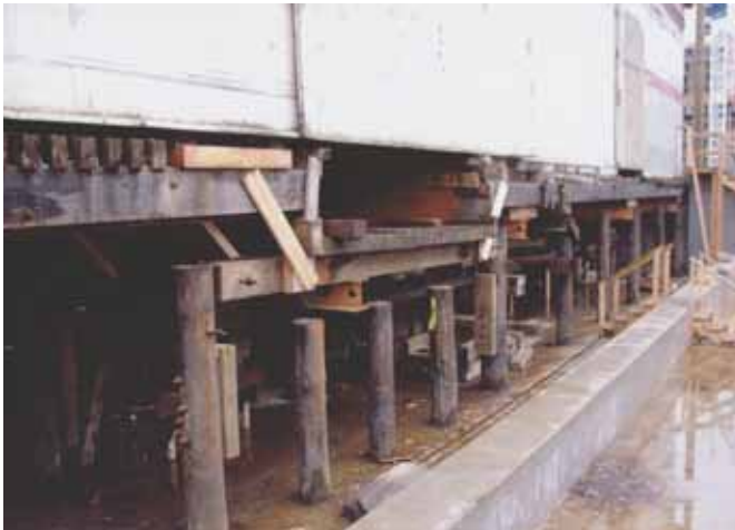
After the first lift
