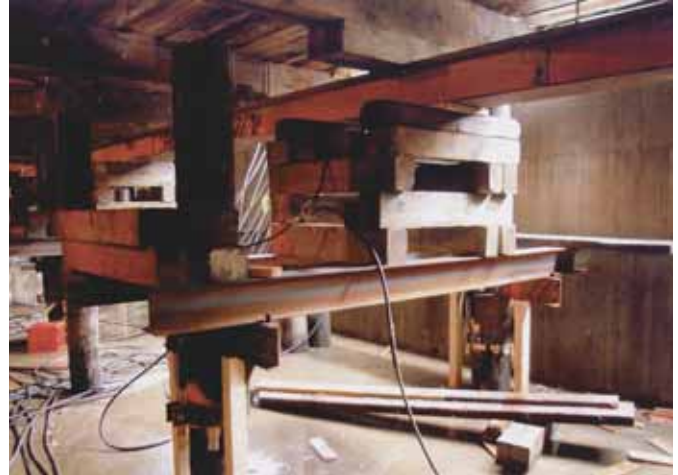
Pile clamps designed for use in the lifting process
