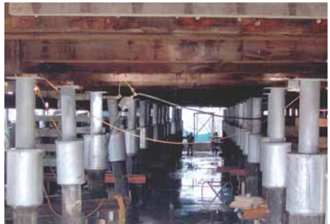
View of pile extensions in place...ready for lowering.
