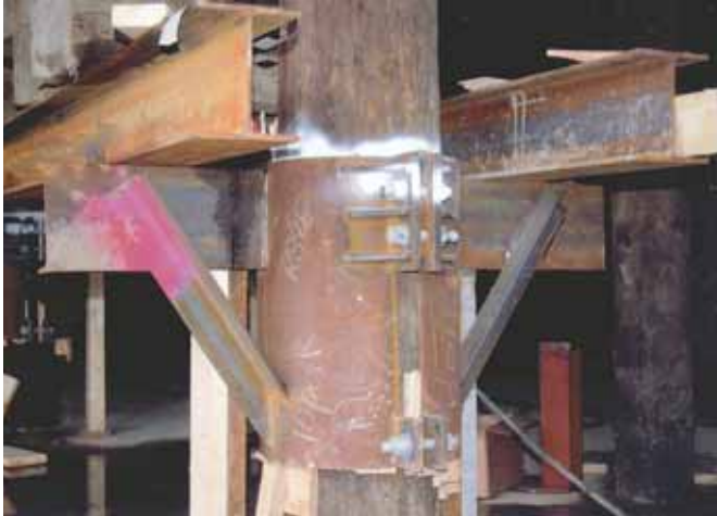
Shows support cribs supported by pile clamps
