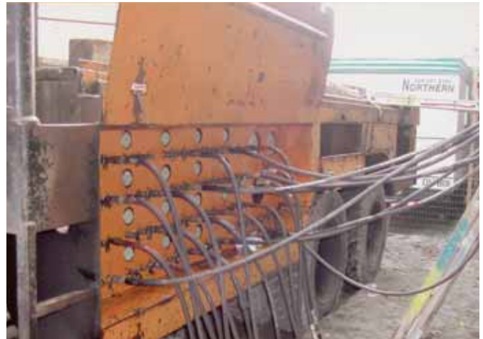
Original Unified Jacking System built around 1956 used to raise Salt Shed
