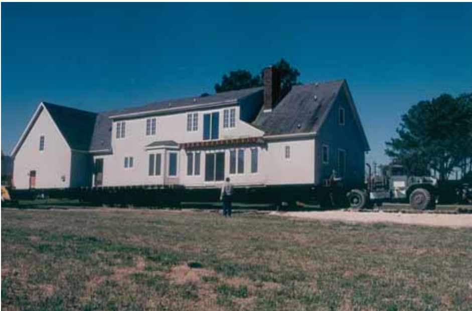
This building was moved out of the fly zone at the Elizabeth City, NC US Coast Guard Base in 1997.
