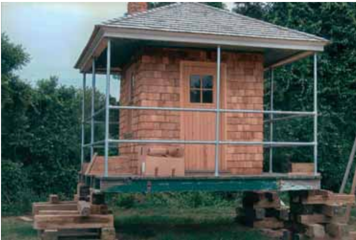
In July 2009 this World War II look-out tower was salvaged and removed from the historic Wash Wood Life Saving Station
