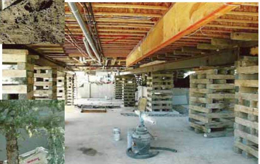
An underside perspective of the length and the crib piers required.
