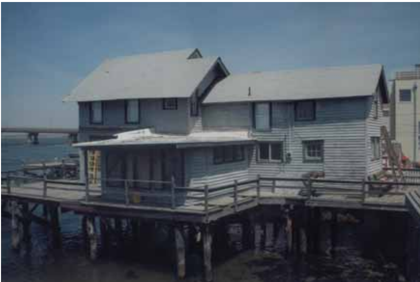
The house before the project began
