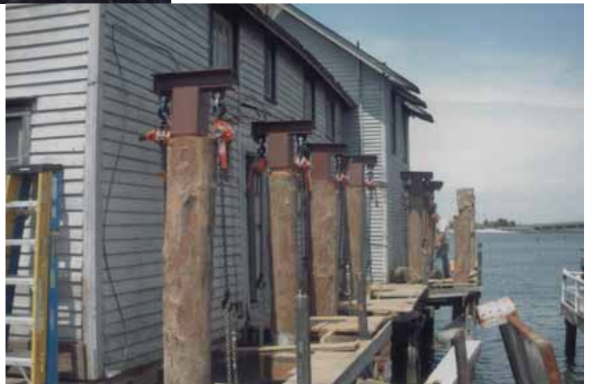
Everything in place and ready to raise
