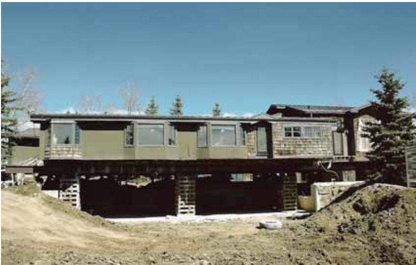
The 117-foot long building was lifted off a walk-out basement
