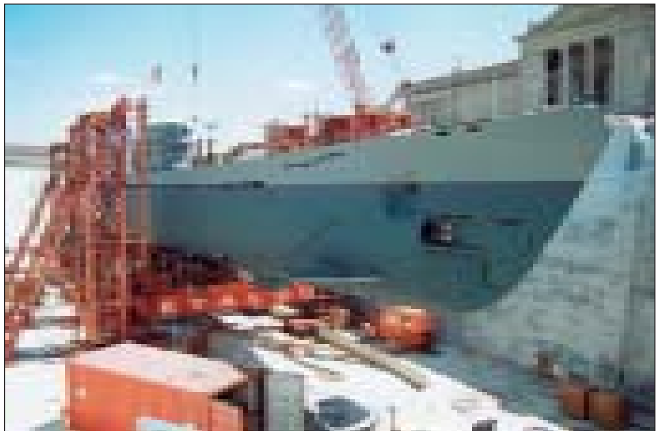
Submarine lowered halfway into the pit of its new home.
