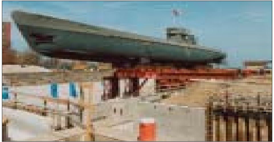
Submarine has been skidded over the pit for lowering.
