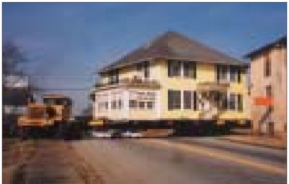
This structure, 40'W' x 60'L was moved three blocks for the City of Wallhalla, SC.
