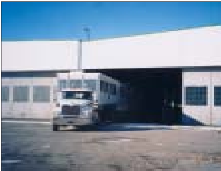
Backing into the new hanger.
