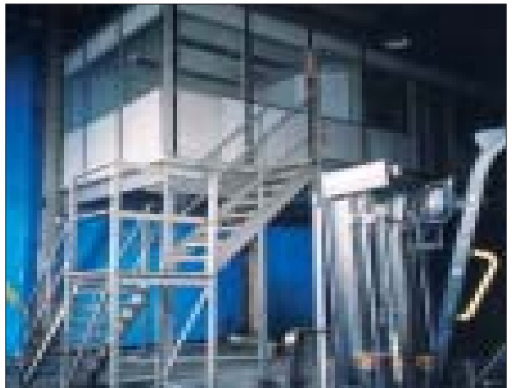
Building in new location.
