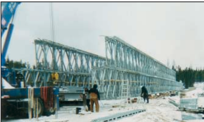
Half-erected bridge being winched and assembled simultaneously.
