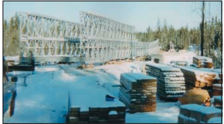
1/4 of bridge assembled and winched.
