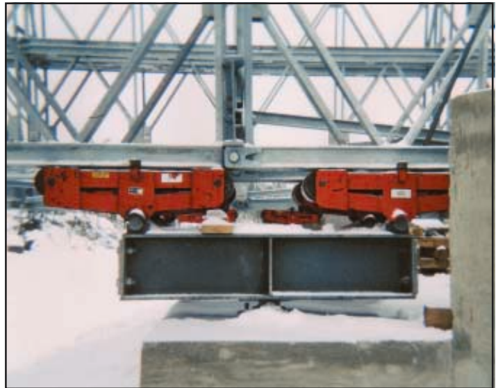
Rocking roller assembly on south abutment.
