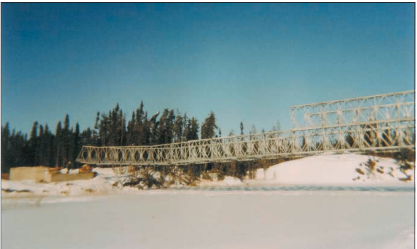
Leading end off bridge with erection nose.
