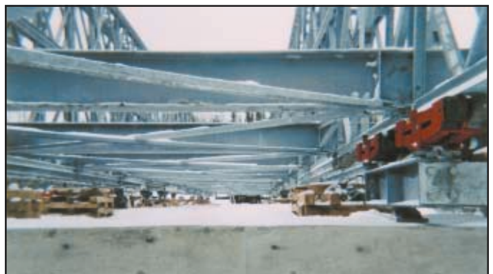
Underside of bridge set up with all rollers on place.
