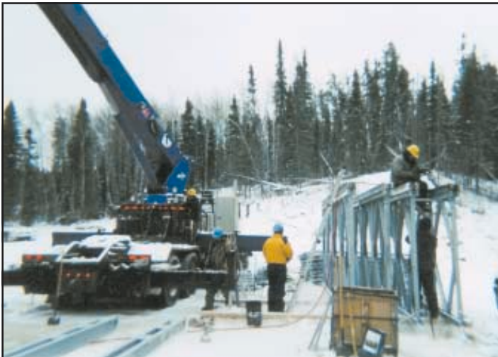
Assembly of parts with our 30T picker truck.
