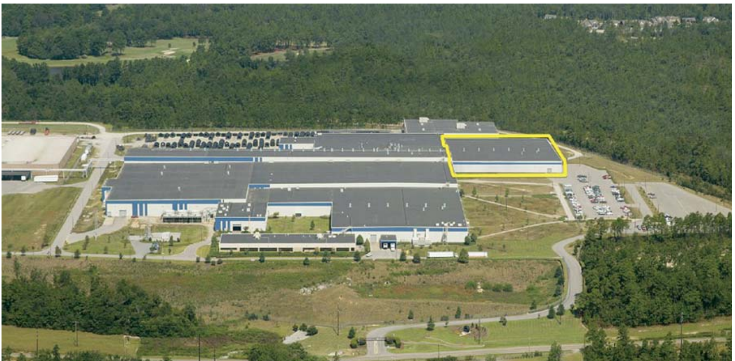
The area above outlined in yellow is part of the $100 million investment Michelin is making at its Earthmover facility in Lexington, SC. The area will contain new curing presses for the company's large mining tires. The company offers 110 different sizes and 45 different tread designs.
