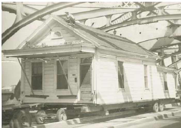
In 1958 this structure was moved on single wheel dollies with a light pull truck. Haywood is on the roof. The bridge is on the I Street Bridge that connects Sacramento with West Sacramento.
