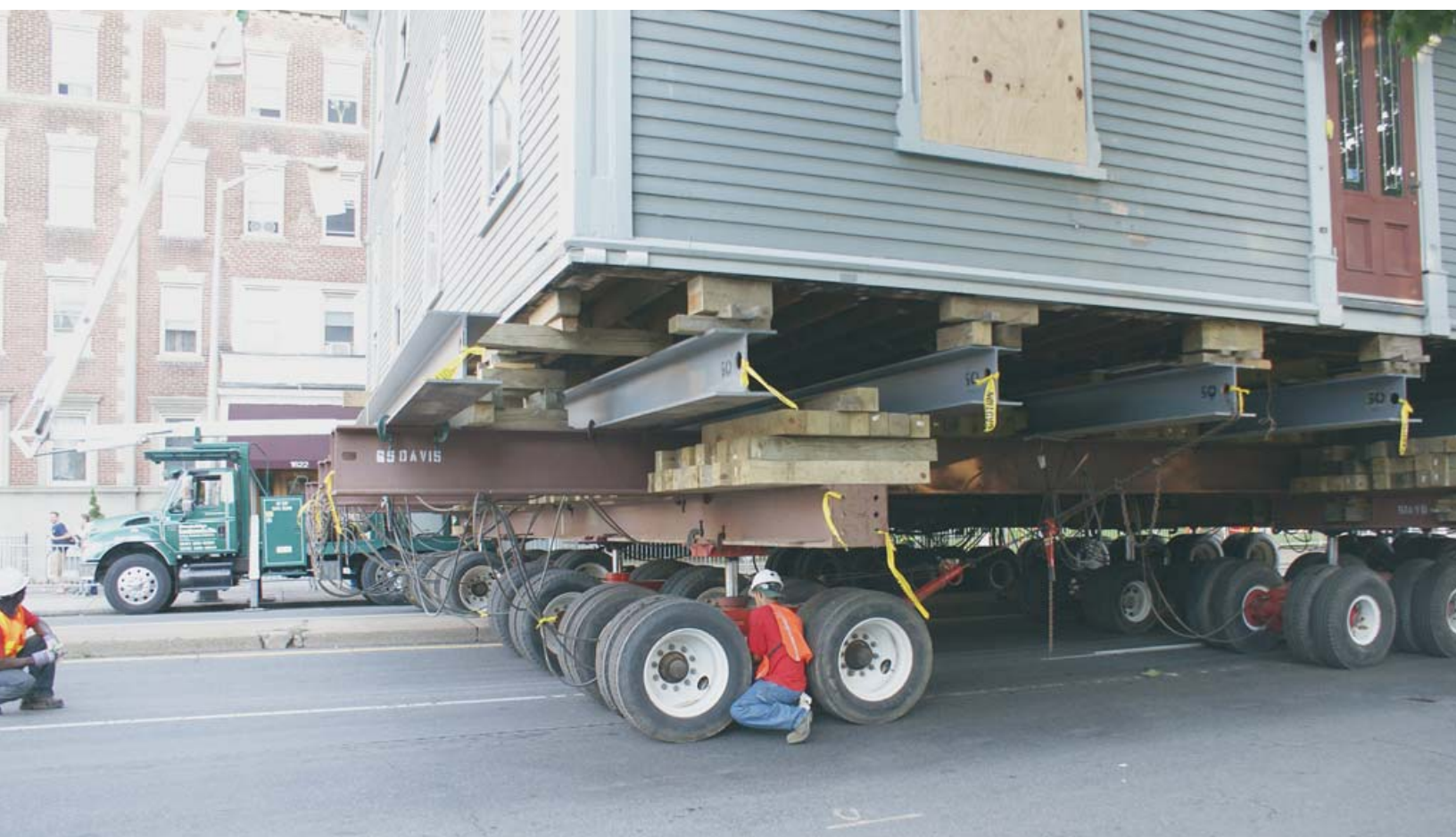
12 dollies, three of which were self-propelled, were used to move the Ukraine House.
