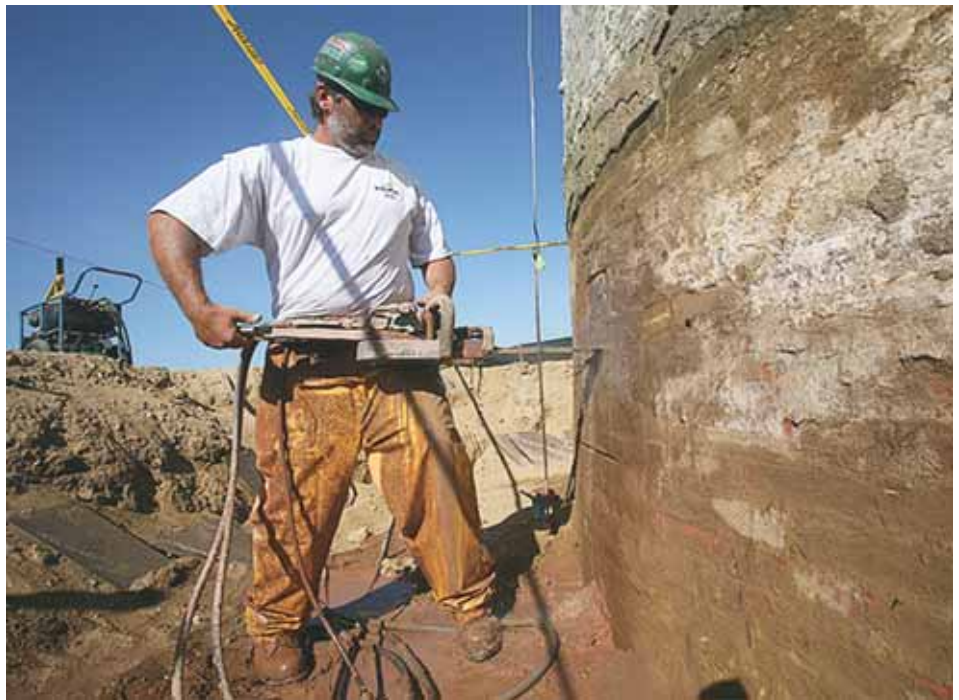
International Chimney employee, John Mitchell, using a hydraulic powered diamond chain saw to cut pocket holes in the original foundation for placement of steel beams.
