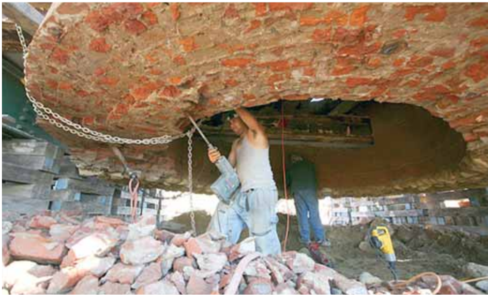
International Chimney employee, John Mitchell, using a hydraulic powered diamond chain saw to cut pocket holes in the original foundation for placement of steel beams.
