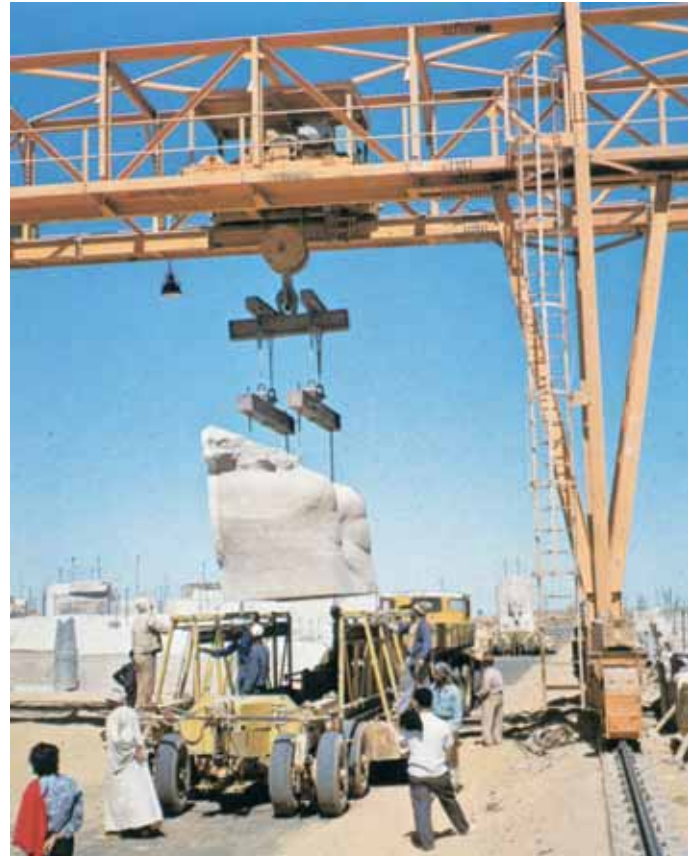
Relocating required cutting the temple into 1,050 blocks, each weighing up to 30-tons. Trucks moved each block 800 meters to a special storage area.
