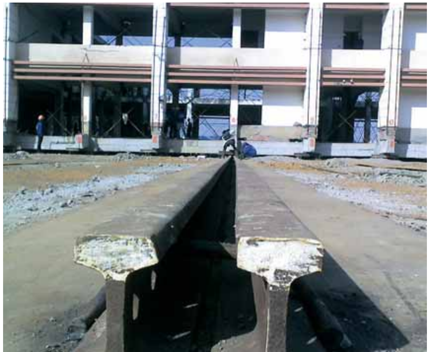
Six rails of 55 meters each, a total of 330 meters, were used. The weight of each rail was 2,150kg for a total of 12,900kg.
