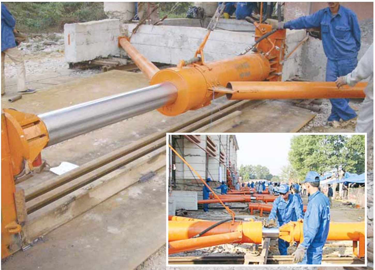
Six rails of 55 meters each, a total of 330 meters, were used. The weight of each rail was 2,150kg for a total of 12,900kg.
