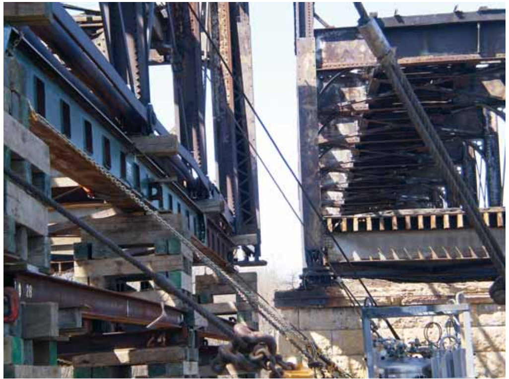
Bridge section being raised off footing to be moved downstream.
