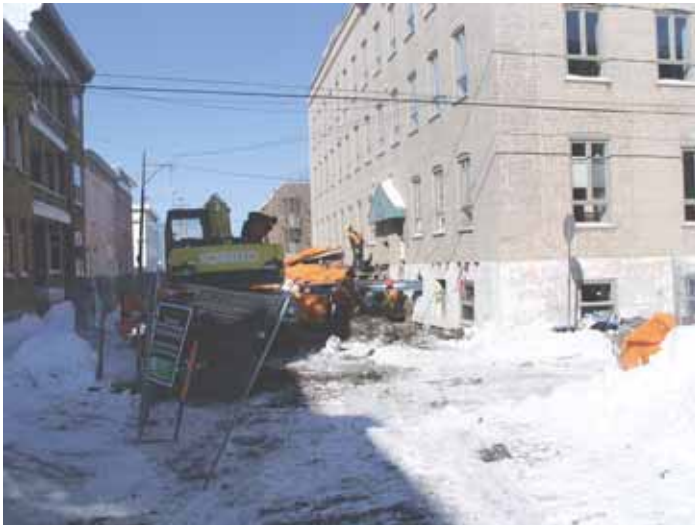
Work was carried out in the dead of winter.
