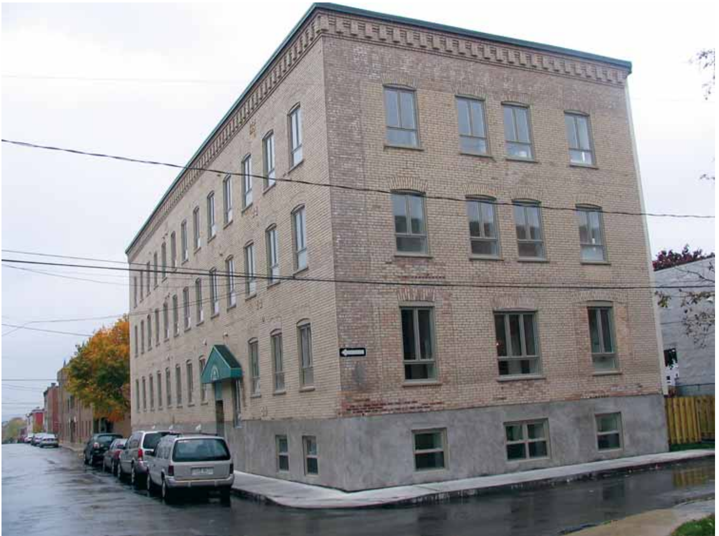
The building with its new foundation.
