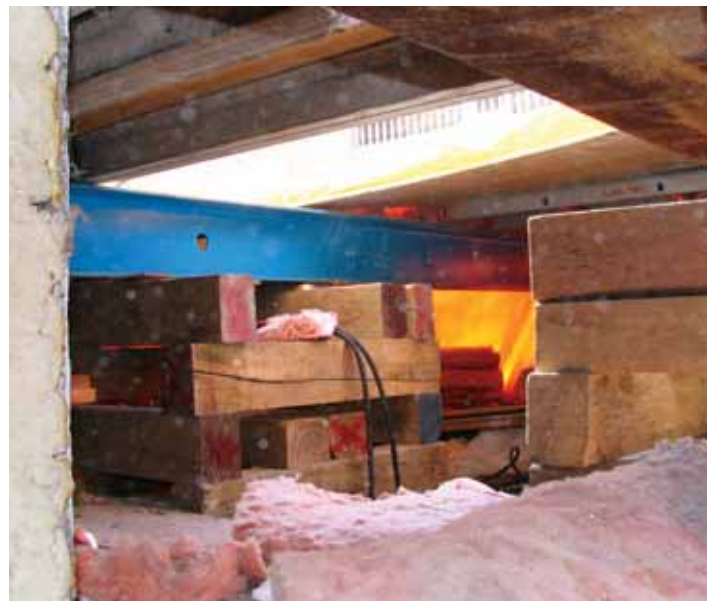
Another view of the shoring equipment.
