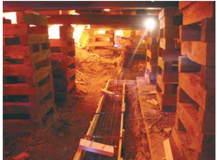
The forms for the new concrete footings.
