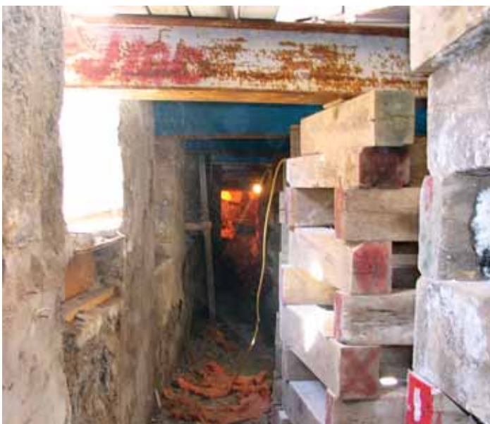
Part of the shoring equipment.
