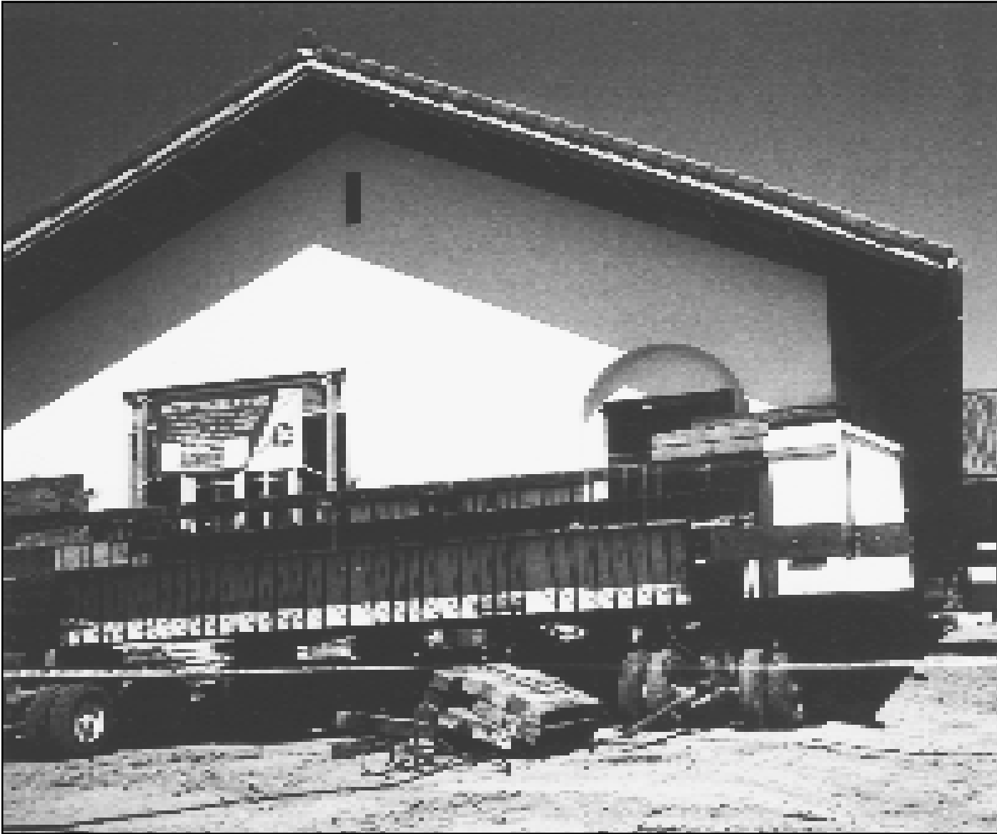
The dolly change complete, the building is now ready to travel to a new location.
