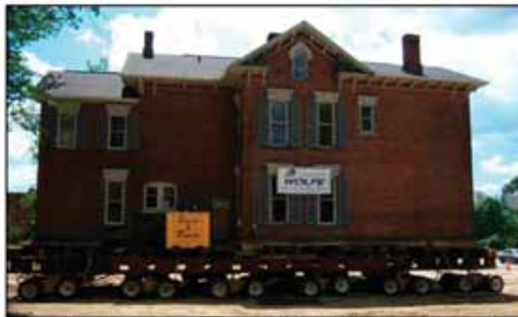
525 ton, triple brick house moved with the Buckingham Power System
